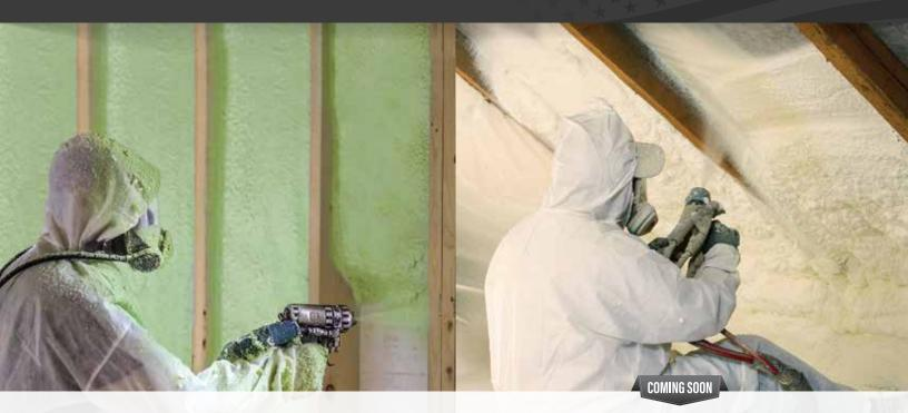
ELITE 2.0 Closed-cell, medium density HFO blown spray foam
