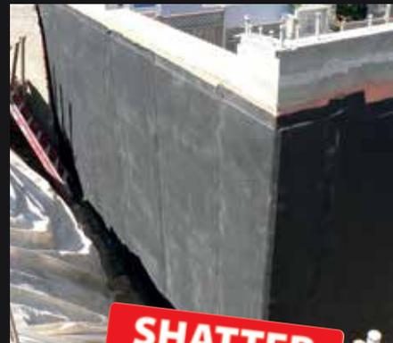
For relief of hydrostatic pressure in vertical foundation applications.
