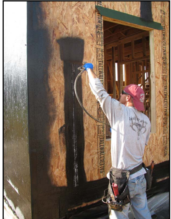
Step Four: Coat fabric with membrane to finish seam
