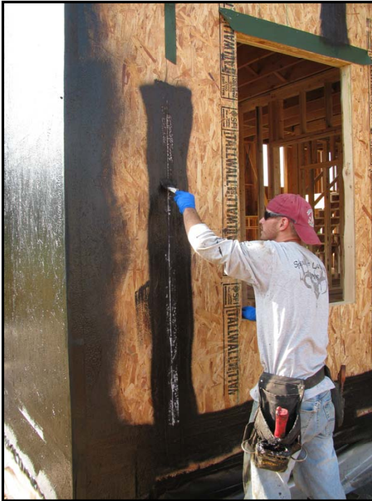
Step Three: Embed fabric into membrane to seat completely
