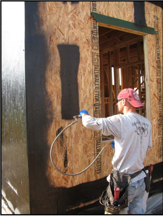
Step One: Coat seam with membrane
