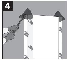
Apply 3M<sup>™</sup> Ultra Conformable Flashing Tape 3015UC in the corners, extending over the vertical sides of window flashing and directly to the wall. Ensure tape is applied with a 2<sup>™</sup> minimum overlap in all directions.
