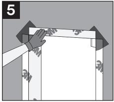
To complete the window detailing, cut a piece of  $3M^{\text{\tiny W}}$  Air and Vapor Barrier 3015 the same width as the window. Overlap a minimum of 2" onto the wall and over the  $3M^{\text{\tiny W}}$  Ultra Conformable Flashing Tape 3015UC in the upper corners.
