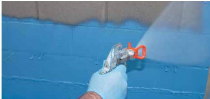
Spray application of Fire Resist Barritech NP60.
