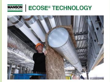
The bonding agents found in traditional fiberglass insulation include nonrenewable petroleum-based chemicals such as phenol, formaldehyde, acrylics and artificial colors. While these materials have little to no impact on the R-value (the ability to resist heat flow) of the end product, they can have adverse effects on the environment.
