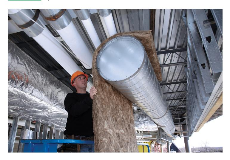
The bonding agents found in traditional fiberglass insulation include nonrenewable petroleum-based chemicals such as phenol, formaldehyde, and acrylics. While these materials have little to no impact on the R-value (the ability to resist heat flow) of the end product, they can have adverse effects on the environment.
