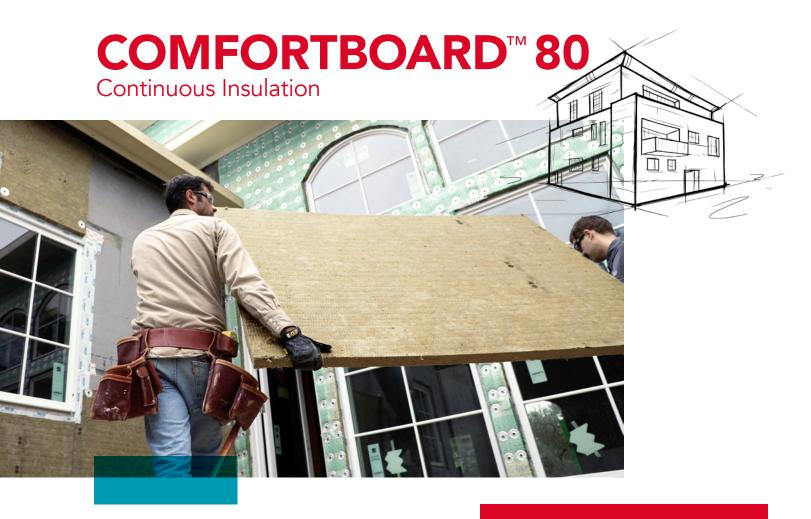
ROCKWOOL COMFORTBOARD™ 80 is a rigid stone wool continuous insulation board used as a non-structural sheathing product in residential construction.
