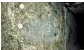
Result w/ Fibrous: Mold growth on insulation
