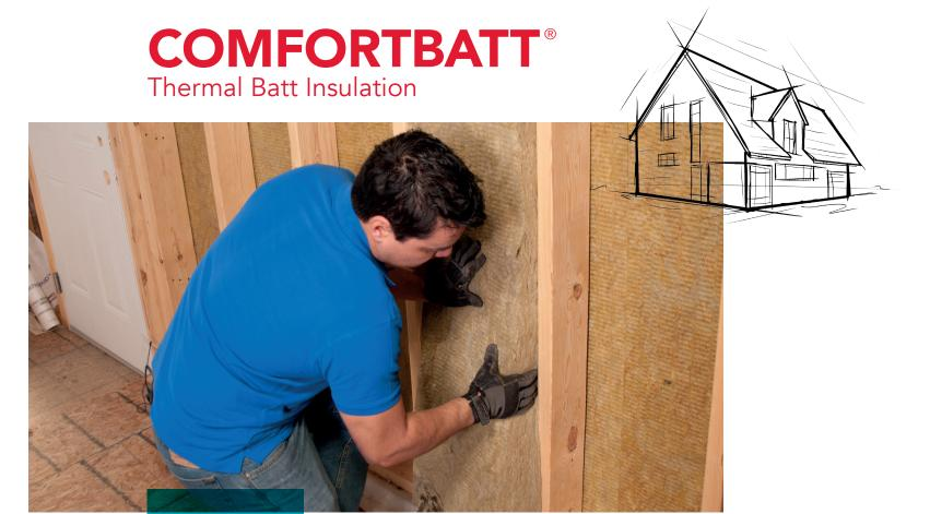
ROCKWOOL COMFORTBATT® is a semi-rigid stone wool batt insulation for exterior wood and steel stud applications in both new construction and renovations.
