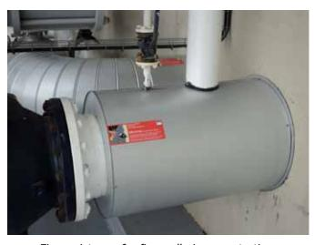
Fire resistance for fire-wall pipe penetrations
