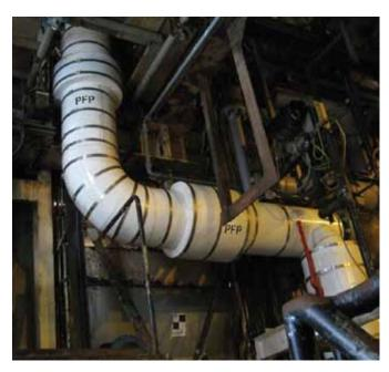
FOAMGLAS® XP: up to two hours of jet-fire resistance
