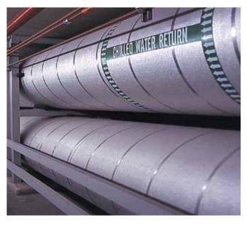
There is simply no other insulation system available in the market today which combines physical strength, fire resistance and moisture resistance to provide the safety and security superiority in chilled water pipe insulation performance.
